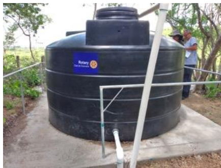
Water tank being installed
