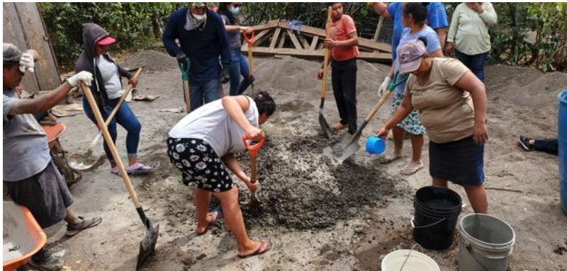
Villagers mixing cement for the new Community Centre
