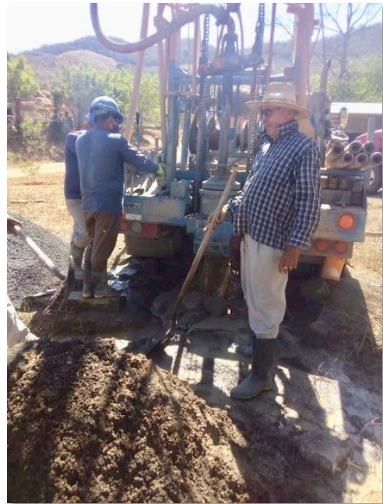
Drilling started in village of El Javillo
