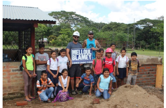
COMMIT Team worked along side the villagers to complete the Community Centre addition
